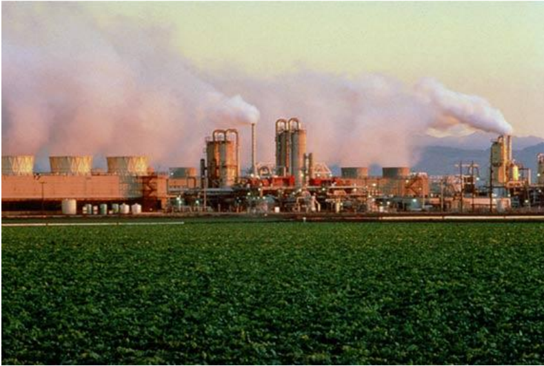
Figure 20: Imperial Valley Power Plant Next to Productive Farmland
