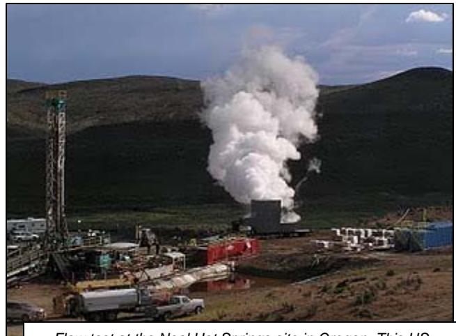
Flow test at the Neal Hot Springs site in Oregon. This US Geothermal project received the first loan guarantee for geothermal technologies under the DOE program. Photo: US Geothermal
